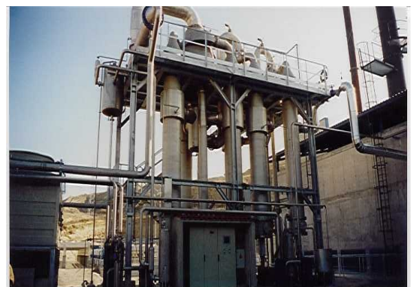
Evaporator for the RO concentrate
